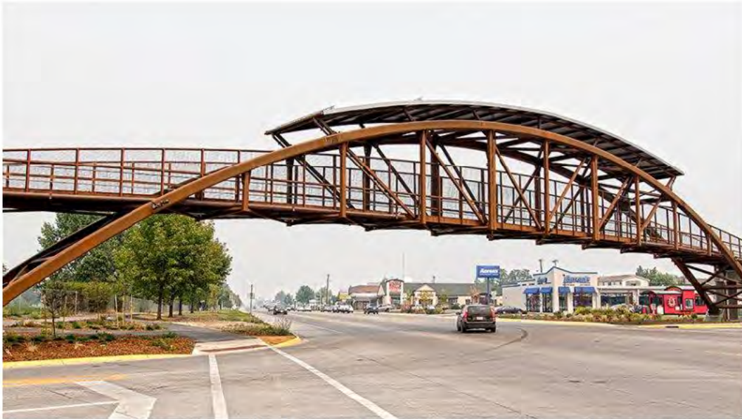
Figure 6.1-12 Pont piéton de la rue South Reserve Street ou le ( http://www.dci-engineers.com/project/reserve-street-pedestrian-bridge )
