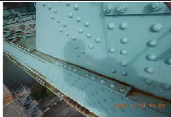
Photo 1: Face amont JC_6_161024_EM_1396
