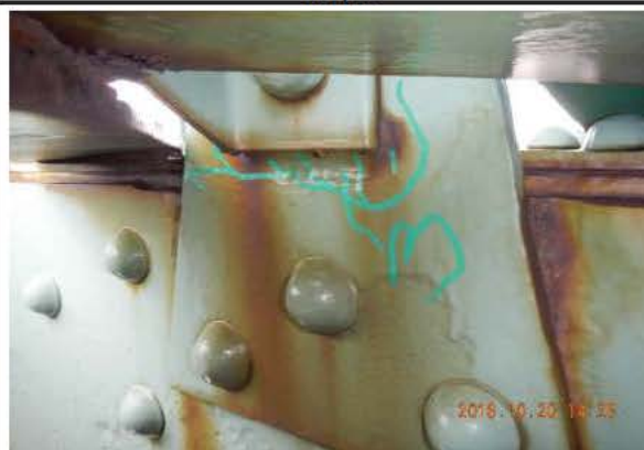
Photo 2: Face aval JC_6_161020_JM_2060
