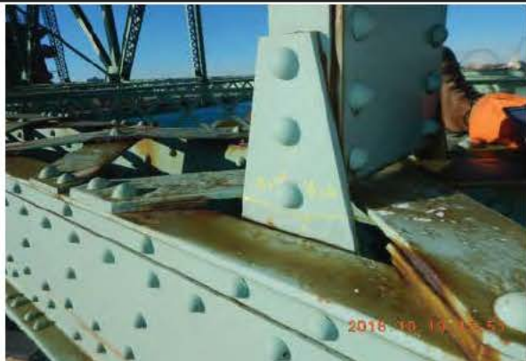
Photo 1: Face amont JC_6_161019_EM_1275
