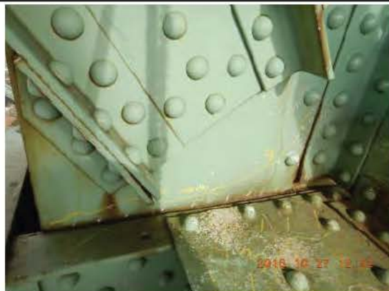
Photo 1: Face amont JC_6_161027_MB_1257
