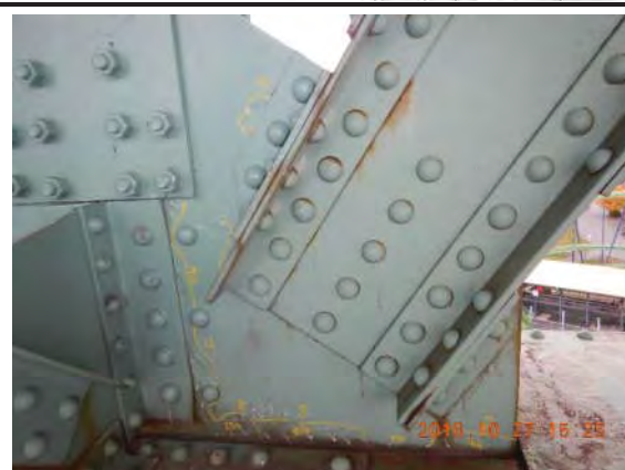
Photo 2: Face amont JC_6_161027_EM_9033
