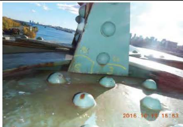
Photo 2: Face aval JC_6_161019_EM_1276
