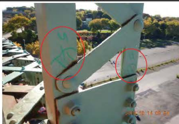
Photo 2: Face nord JC_6_161014_JM_1937
