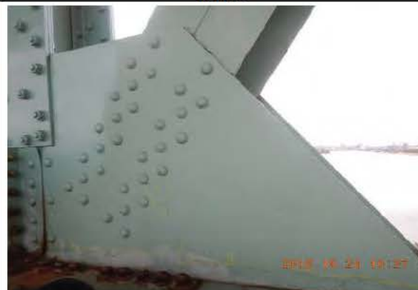
Photo 2: Face aval JC_6_161024_EM_1402
