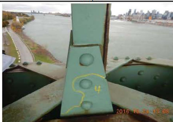
Photo 2: Face aval JC_6_161024_EM_1441
