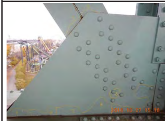
Photo 1: Face amont JC_6_161027_EM_9032
