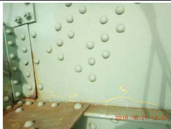
Photo 2: Face amont JC_6_161027_MB_1256
