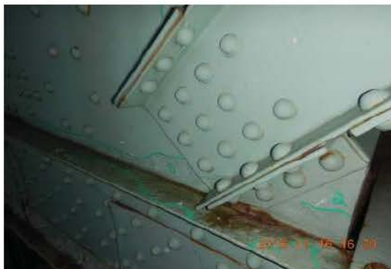
Photo 1: Face amont JC_6_161116_EM_9858
