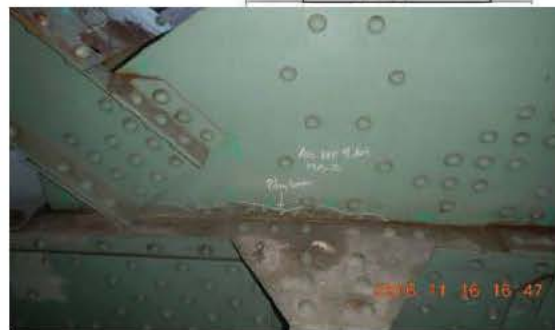
Photo 2: Face aval JC_6_161116_EM_9861
