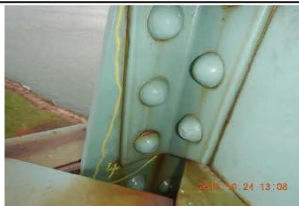
Photo 1: Face amont JC_6_161024_EM_1439
