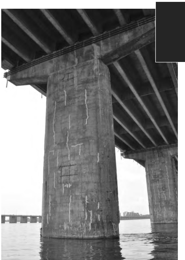
S5.PC.2.2.a – 5001 - Pile 13W (face est)
