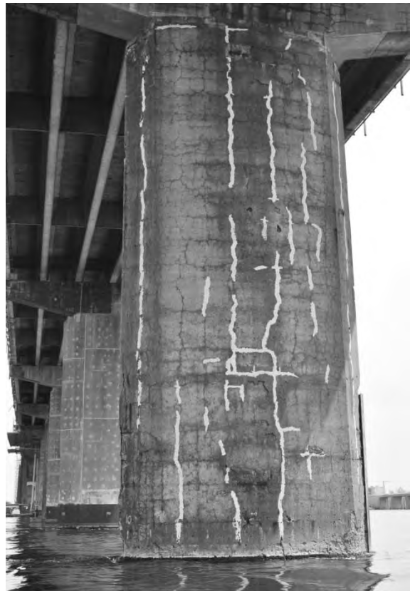
S5.PC.2.4.b – 5012 - Pile 11W (face ouest)
