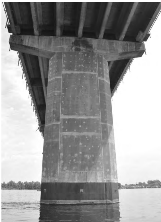
S5.PC.2.6 – 5028 - Pile 9W
