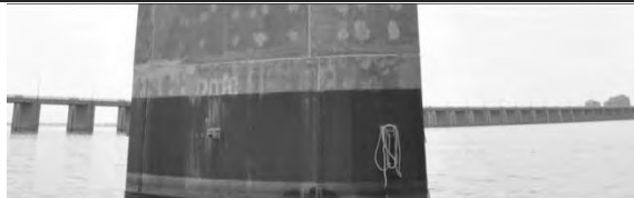
S5.PC.2.10.a – 5061 - Pile 5W (face est)
