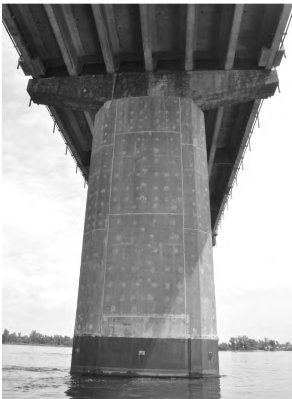
S5.PC.2.5 – 5021 - Pile 10W
