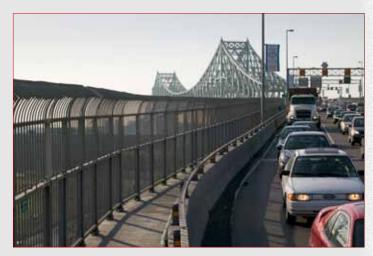
The Bridge is in relatively good condition however the bridge is now over 80 years old and certain elements will require repairs in the next few years, notably repairs to the piers, replacement of bearings, repairs to certain steel components and renewal of the roadway pavement and painting.
