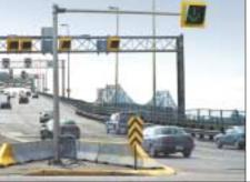
Closed-Circuit Television Surveillance System cameras and lane signalling on the Jacques Cartier Bridge.
