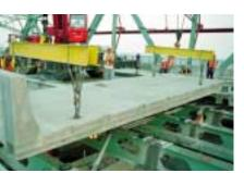
Installation of a deck panel in roadway
