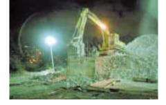
Demolition of old slabs from bridge, to be recycled as aggregate
