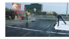
Application of first layer of asphalt
