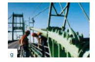
The Seaway International Bridge [f] connects New York State and the Ontario city of Cornwall, passing through the Mohawk community of Akwesasne. The Corporation is conducting annual "hands on" inspections, removing loose material from the underside, and patching the surface. The deck of the South Channel Bridge was re-paved and SIBC crews sandblasted and re-coated the legs of the south main tower.
