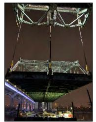
Lowering of the suspended span at night
