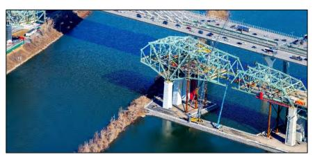
Deconstruction of the steel structure of the Champlain Bridge
